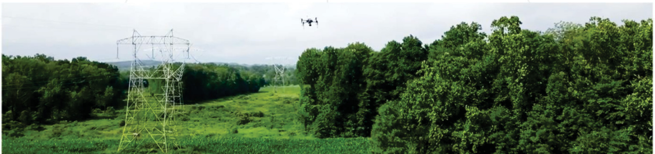
Photo courtesy of First Energy
